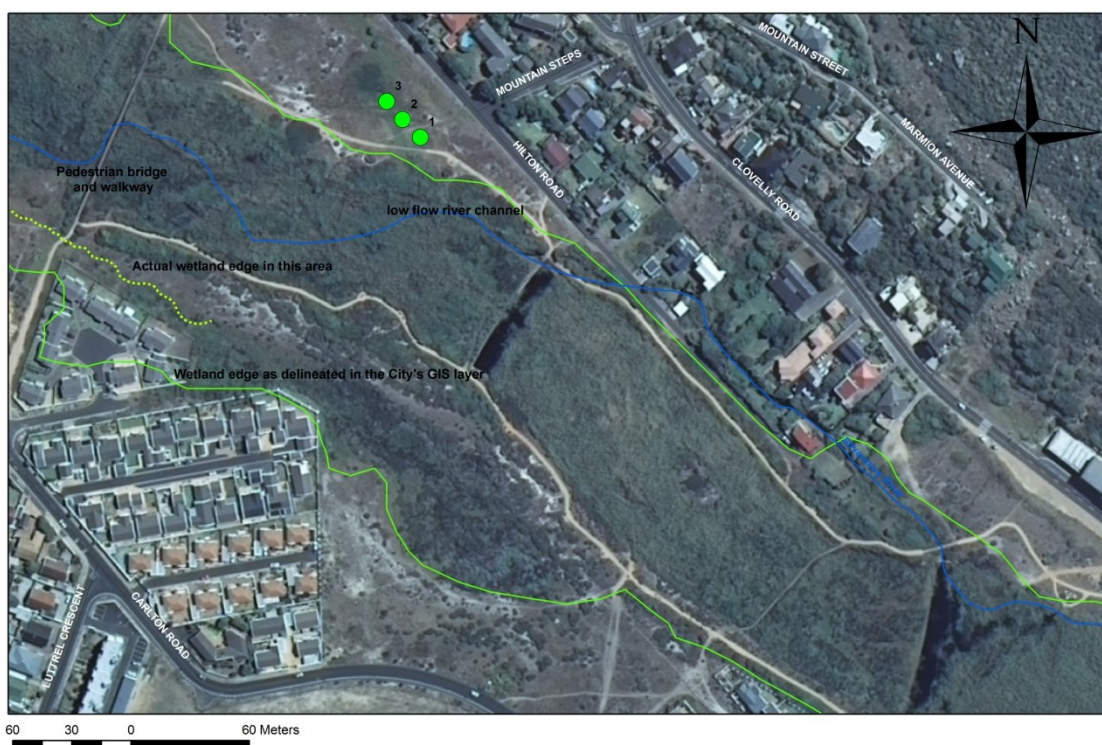
Figure 3 2010 aerial photograph (as in Figure 2) showing wetland extent as per the City's (2009) GIS layer) (unfilled green polygon); river channel (blue line), spot locations (numbered green circles) showing positions of the depressional wetlands (referred to as hillslope seeps in Emms and McDonald (2012) and with dotted green line in the vicinity of the pedestrian bridge showing the revised wetland edge in this area, based on Day (2009)'s delineation in this area and ground-truthing in 2012.
