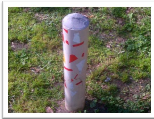
Figure 6. PVC pipe filled with concrete
